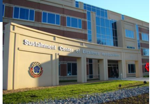
Fort Lee's new Sustainment Center of Excellence is the first major BRAC 2005 project completed on the East Coast. VNDIA photo.
